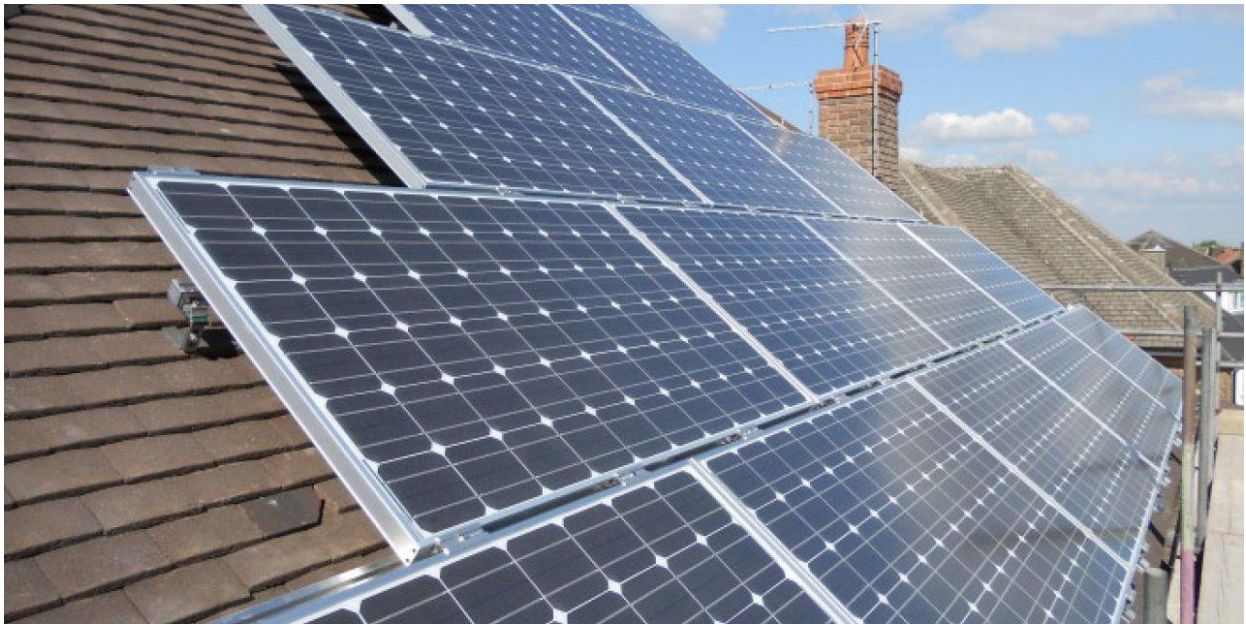
Figure 30: Micro PV installation
